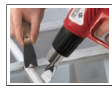
Removal of window glazing
