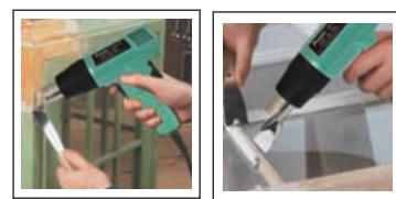
Paint and varnish removal
