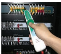
Copper cabling detecting
